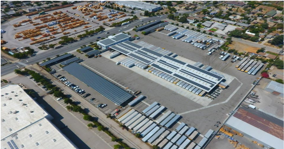
Figure 1: Aerial view of the DHE cross-dock facility in Ontario, California.
