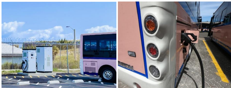
Figure 2: The CCS2 DC charging stations by SSE International at a bus depot in Bermuda.
